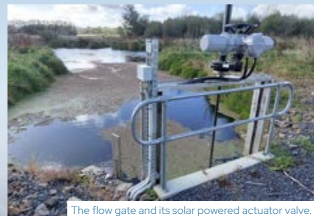
The flow gate and its solar powered actuator valve. Photo: ORC/Tim Ware
