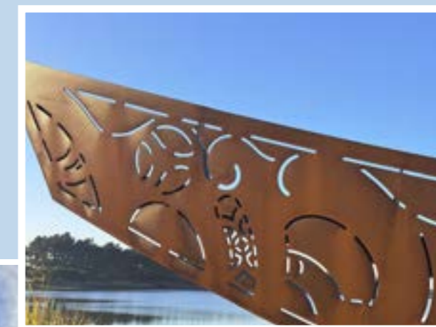
Mahi Toi designs associated with the pump station are integral to the wider Stead Street climate resilience project. The above image shows the design detailing at the end of the new sheet pile wall, conceptually transforming it into a Waka Tiwai.
