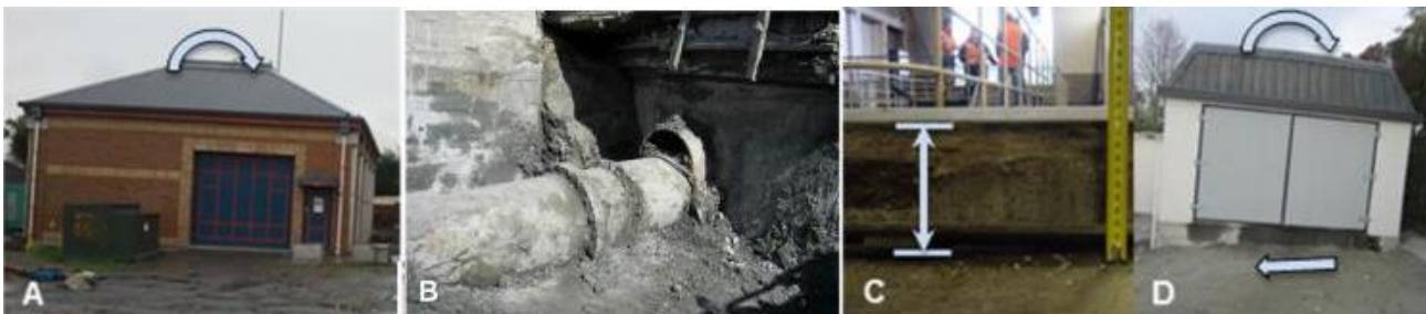
Figure 4: Common failure mechanisms at pump stations
