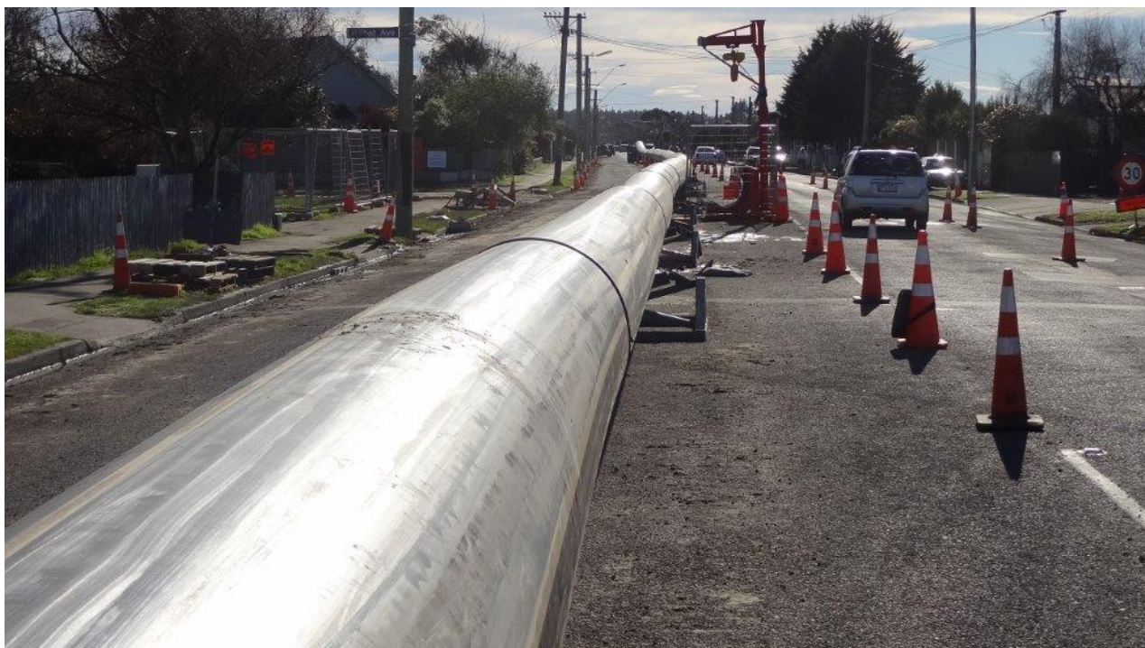
Figure 3: The DN800 PE PM 128 pipe running along Bower Avenue prior to installation by directional drilling.
