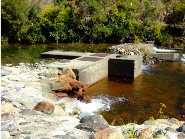
Photograph 5: Intake weir and backfeed discharge, Maitai River
