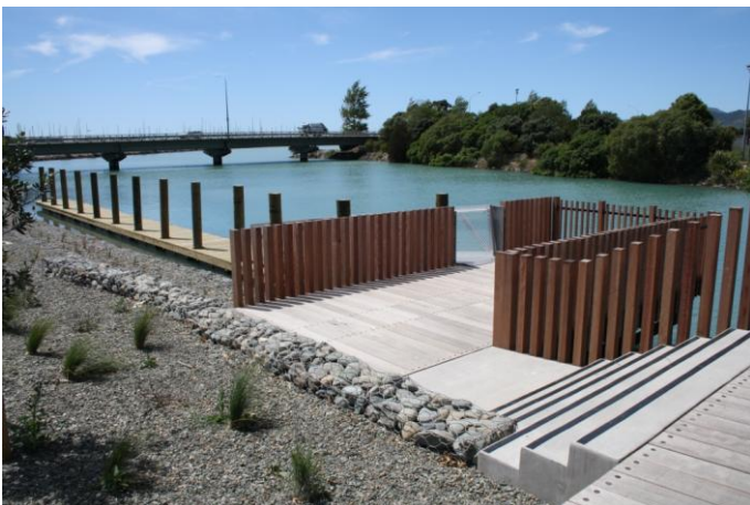
Photograph 8: Maitai Walkway and pontoon development, Nelson
