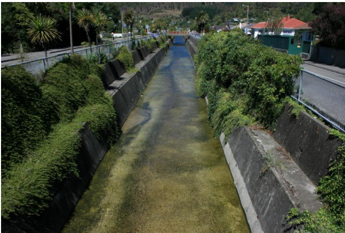
Photograph 6: Brook Stream concrete channel, Nelson
