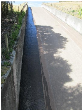
Photograph 10: Spat ropes and wet margin, Maitai Dam Spillway
