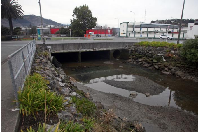
Photograph 7: York Stream culvert, Maitai tributary, Nelson
